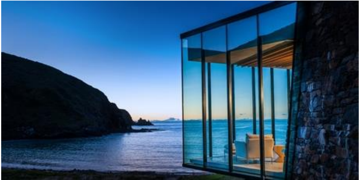
At the end of Annandale's peninsula, stands the ultra-modern, concrete, stone and glass hideaway called 'Seascape' at Whitehead Bay. Photo / Stephen Goodenough
